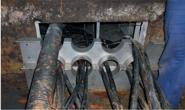
Installation of the pre-mounted flange plate and marking of installation positions in front of the wall entry.
