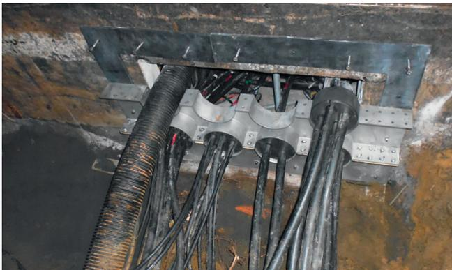
Step by step installation of the flange plate with long-shaft fixing dowels and stainless steel bolts.
