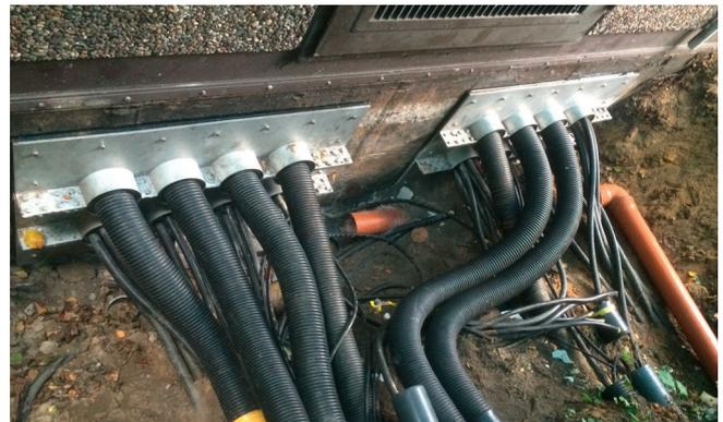
New wall entry with cable and duct ditch before grouting.
