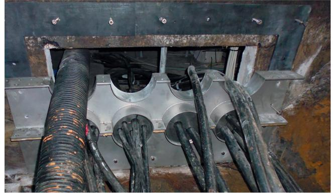
Adhesive bonding of the flat seal via Sikaflex sealing compound.
